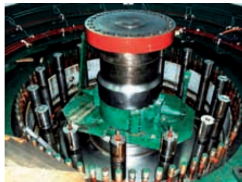
...rotora crpke-turbine 2 i privodnih lopatica
