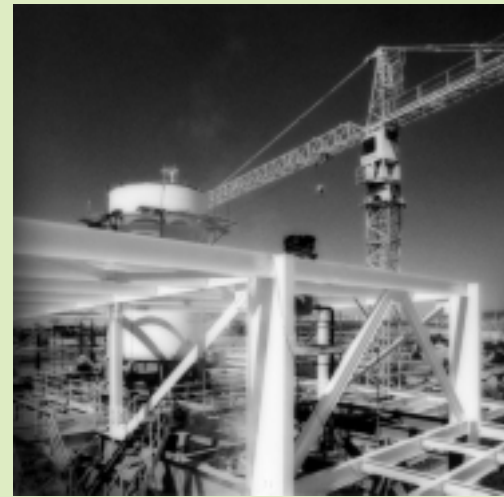
TE-TO Zagreb - construction of the new cogeneration unit
