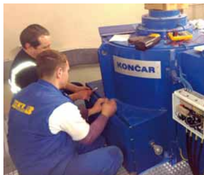
Radovi na generatoru ABM HE Varaždin
