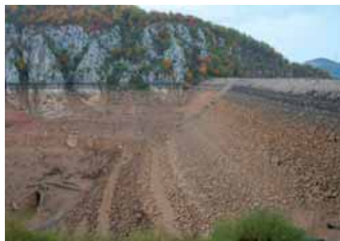
...s druge strane, brana HE Sklope oslobodena težine vode
